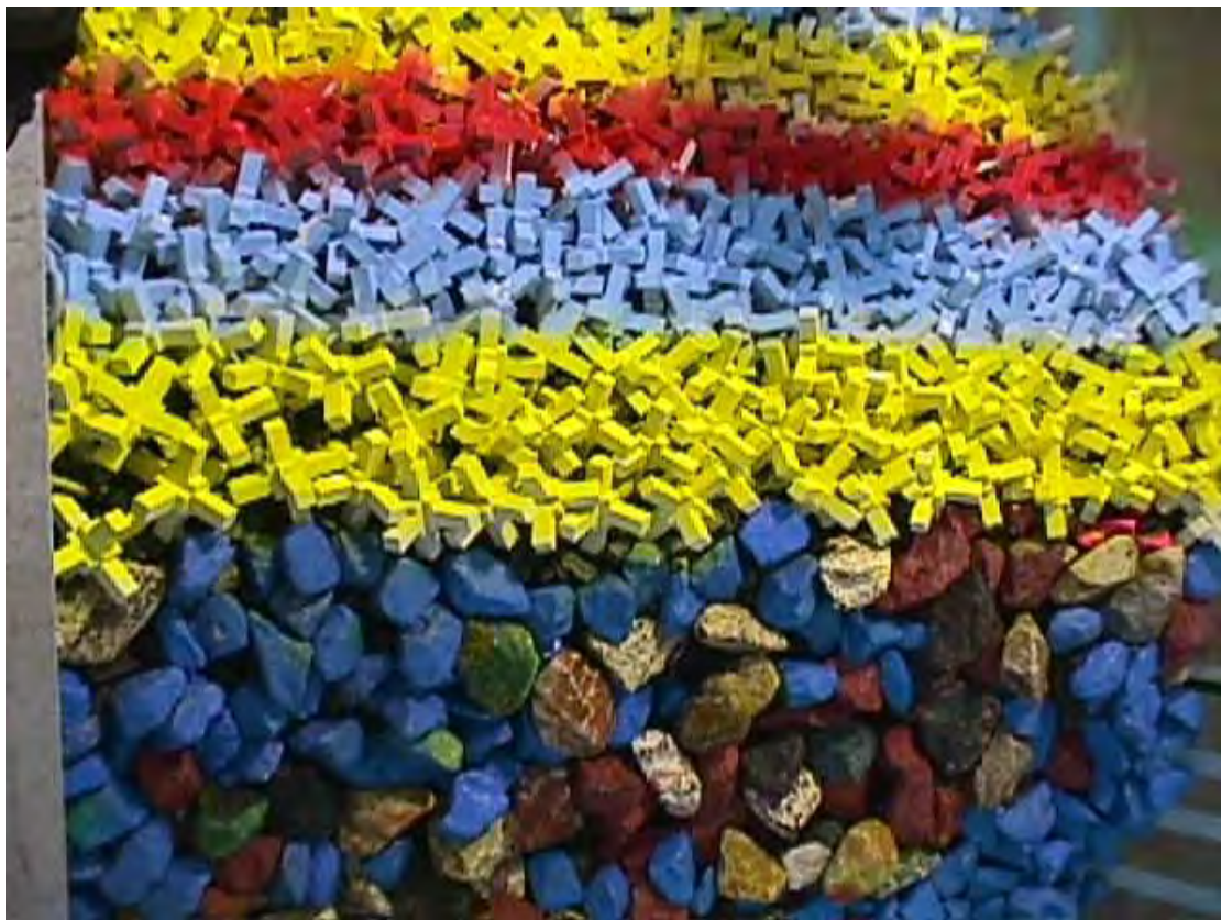
(b) Minor damage to crest after extensive overtopping when using Ajacks units for crest protection H_s 4.5 \text{ m} , T_p = 8.0 \text{ s}
