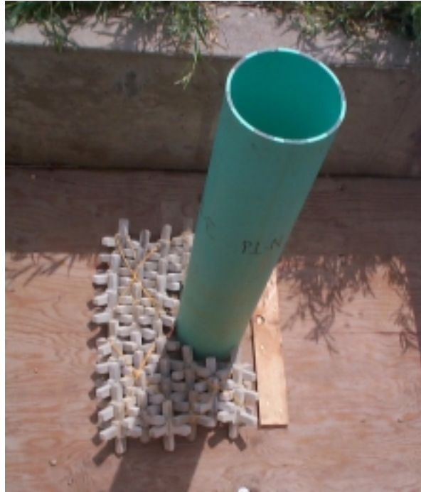
Figure 3.4a. A-JACKS 5x4x5 modules in a typical pier scour installation.
