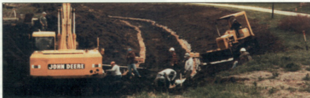
Excavation work progressing.
