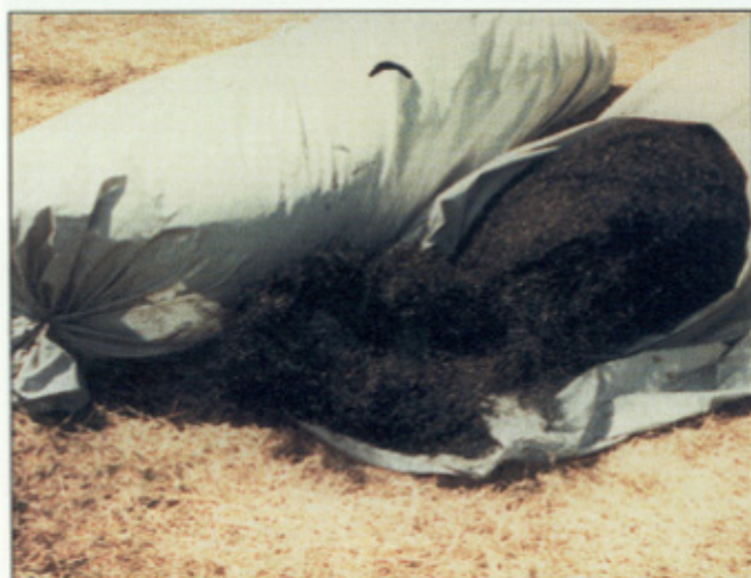
Left: This FiberDam product, which is black geotextile fibers, was placed behind the A-Jacks in order to prevent losing any backfill material back into the channel. Right: The A-Jacks product was utilized instead of rip rap to control the erosion in the Beals Slough project. Andy Bailey, with the Lower Platte River South district, said this was the first application of this product in the area.
