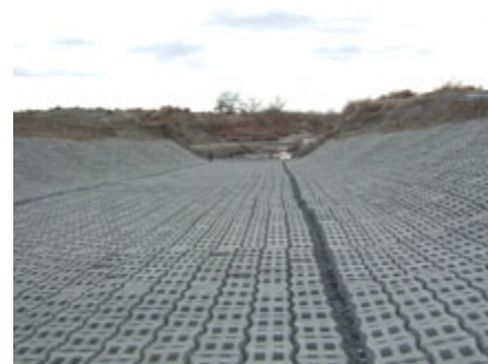
ArmorFlex installation complete
