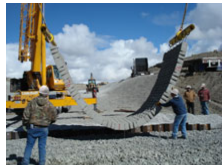
installation of ArmorFlex
