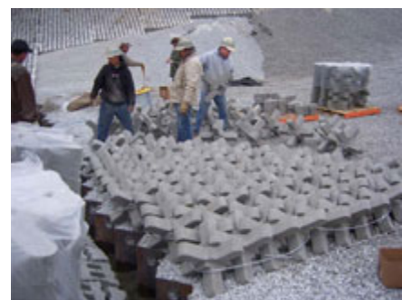
installation of A-Jacks
