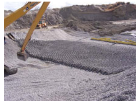
A-Jacks installation complete
