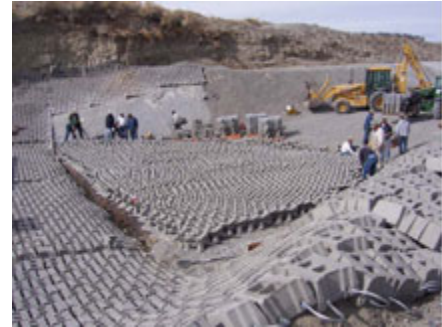
installation of A-Jacks continues
